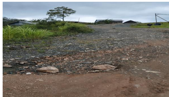
Figure 2. The road to Fatumnasi village (Source: own research, 2024)
